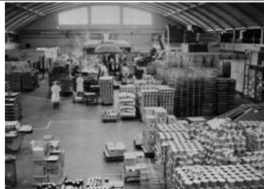
Interior in 1950's / 60's as Marmalade Factory
