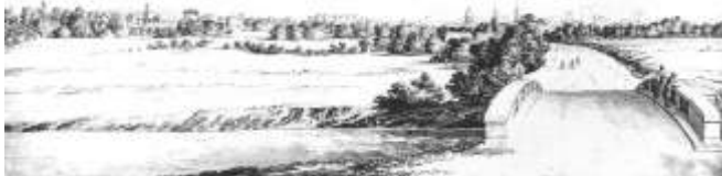
1781 from Bulstake Bridge
