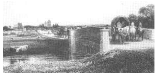
1851 from Seven Arches Bridge (no longer standing, near Lamarsh Road)
